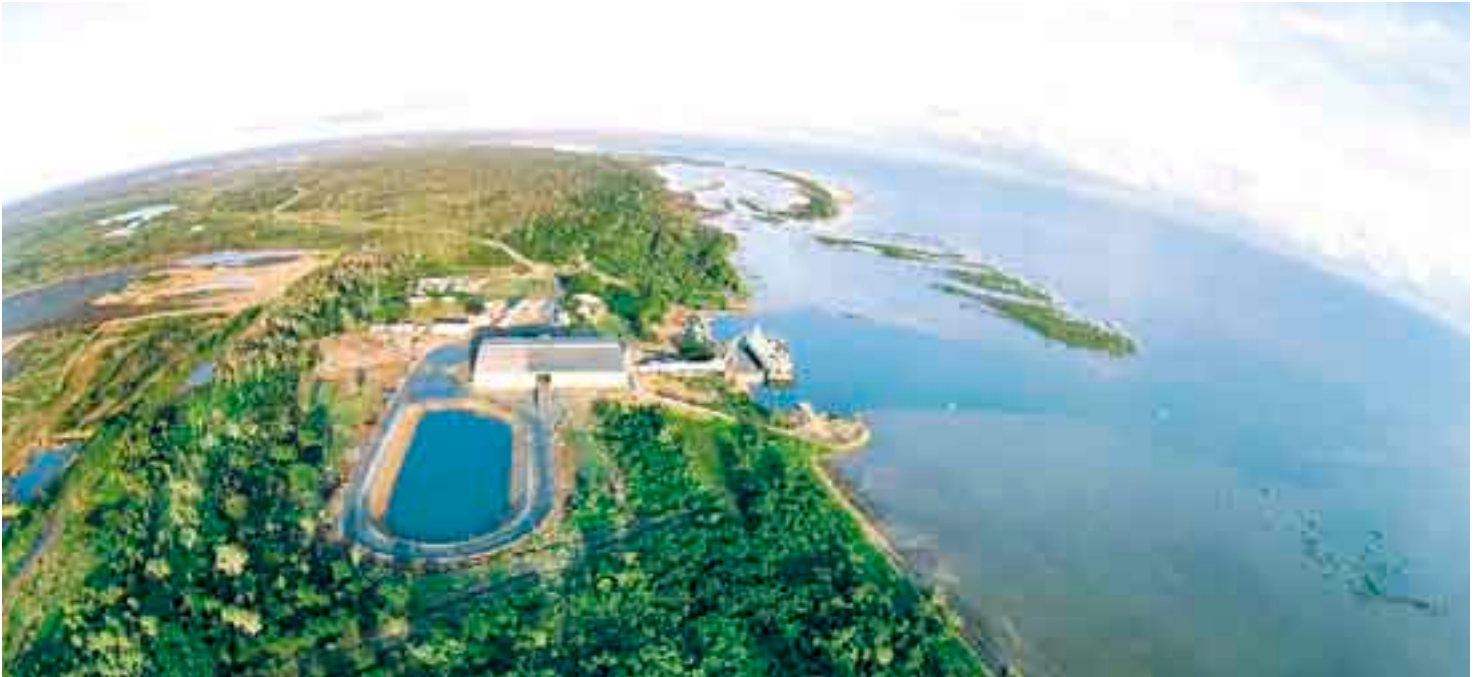
Aerial view of the Bing Bong loading facility.
