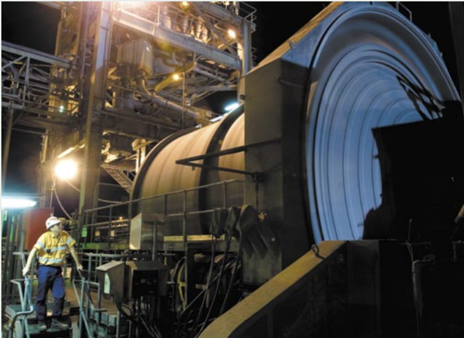
The MRM Processing Plant is a 24 hour operation.
